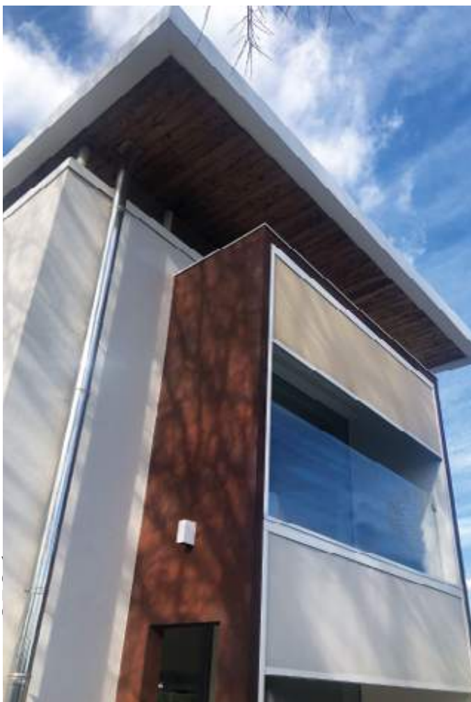
Uffici - Montebelluna (TV) OXYDECOR® Rust / 1 mm. Offices - Montebelluna, Italy OXYDECOR® Rust / 1 mm.
